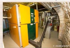
KWB Powerfire 150 - 300 kW
