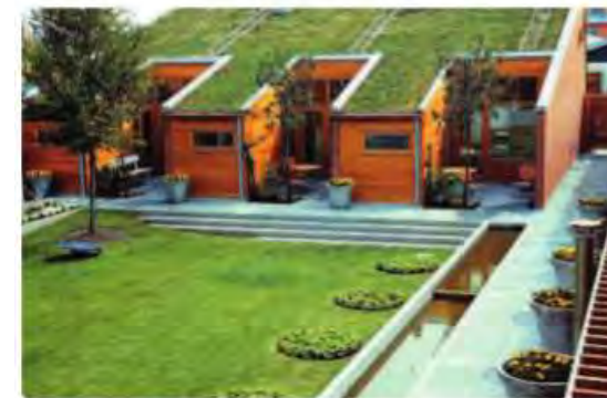
Fig. 4 The courtyard with the highest Green Space Factor (a score 0.84) at Bo01, Western Harbour, Malmö was achieved its rating mainly with mown lawns and sedum roofs
